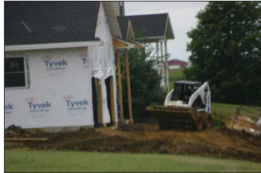
Figure 16. New home construction in Cuba City
